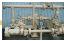
Stop #2 30 psig typical up to 60 psig Metering & Regulator Station
