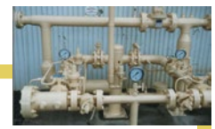
Stop #4 30 psig typical Residential Transfer Station
